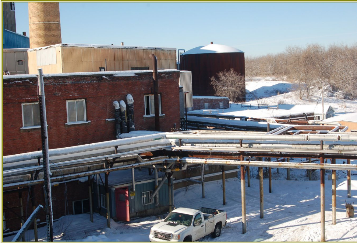
Powerhouse Building #23 Pipe Rack North & East Side
