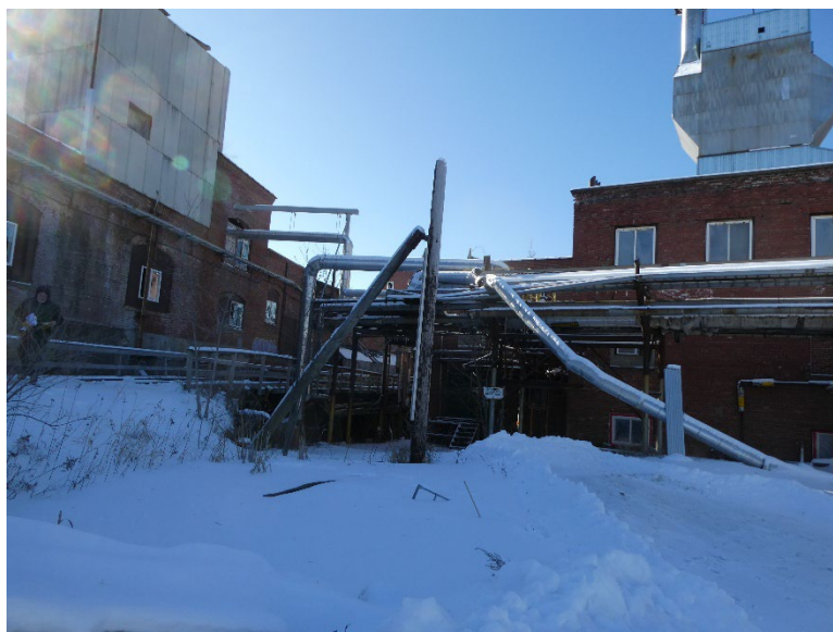
Electrical Pole with angle support to be removed, East Side Building 23
