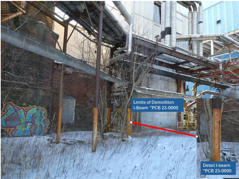
Limits of Demolition, West side
