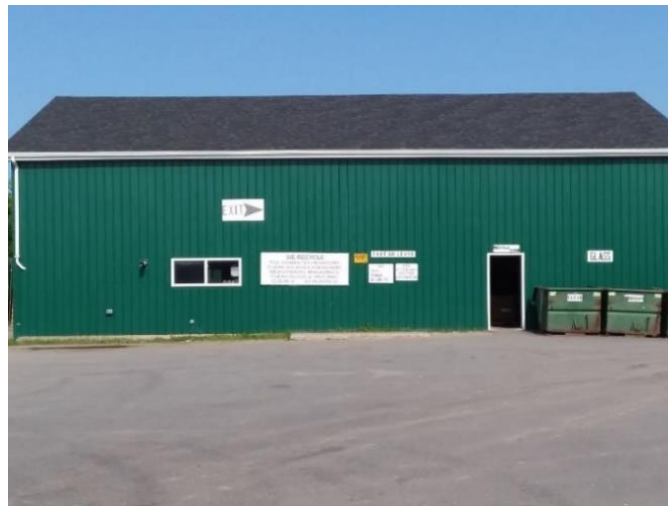
Transfer Station Recycling Center
