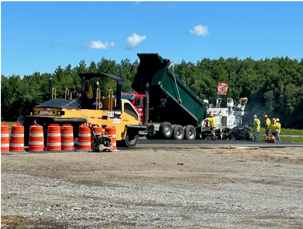
Apron Reconstruction Project
